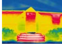
Building: Heat Loss
