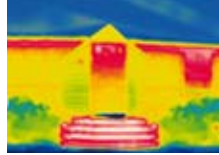
Building: Heat Loss
