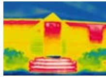
Building: Heat Loss
