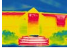
Building: Heat Loss
